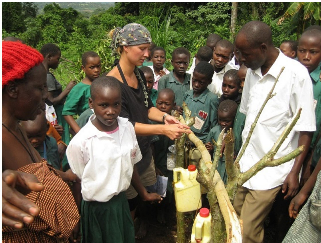
Tina Bartelmeß a volunteer with KWDT works with Kiyoola Primary School to install tippy taps and train School Sanitation Clubs.
