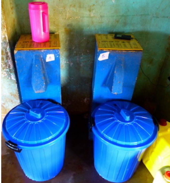
Purification of drinking water at St. Andrews Primary school – Kisoga
