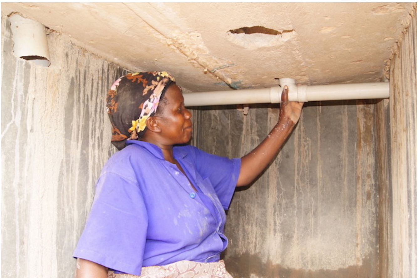
Ms. Lydia Kateregga ; Ecosan manson. Women construct and promote appropriate technologies eg the ecosan toilet ( dry toilet) appropriate in fisher communities with high water table and in rocky areas.
