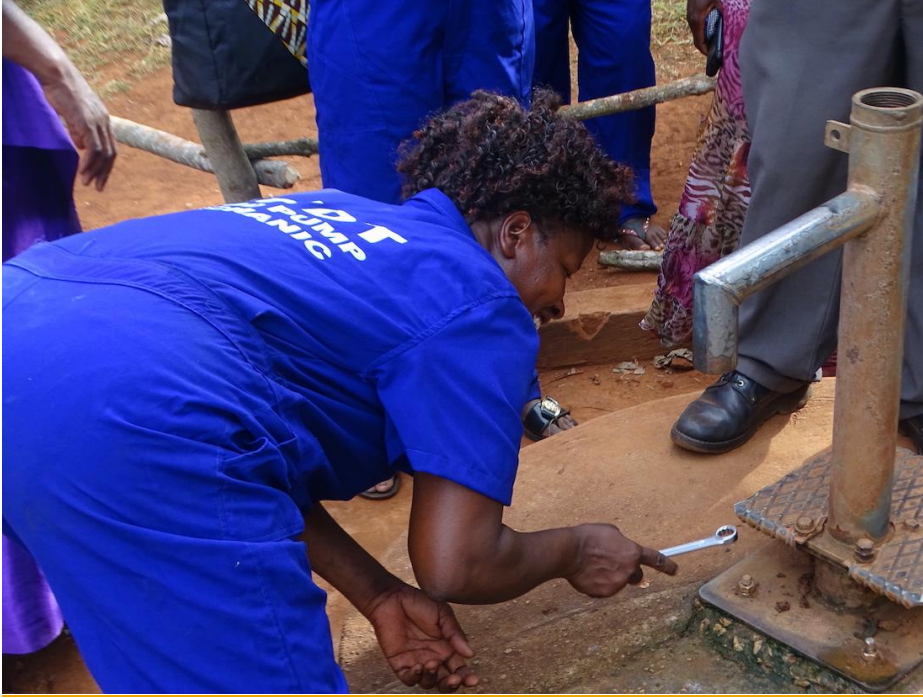
Nantale Harriet, handpump mechanic from Kulubbi Women's Group in Ntenjeru sub county employs skills acquired to repair hand pump wells
