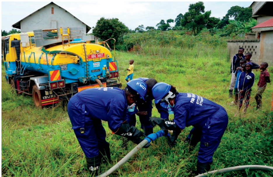
KWDT cesspool operators, two women and one male truck driver, empty a latrine
